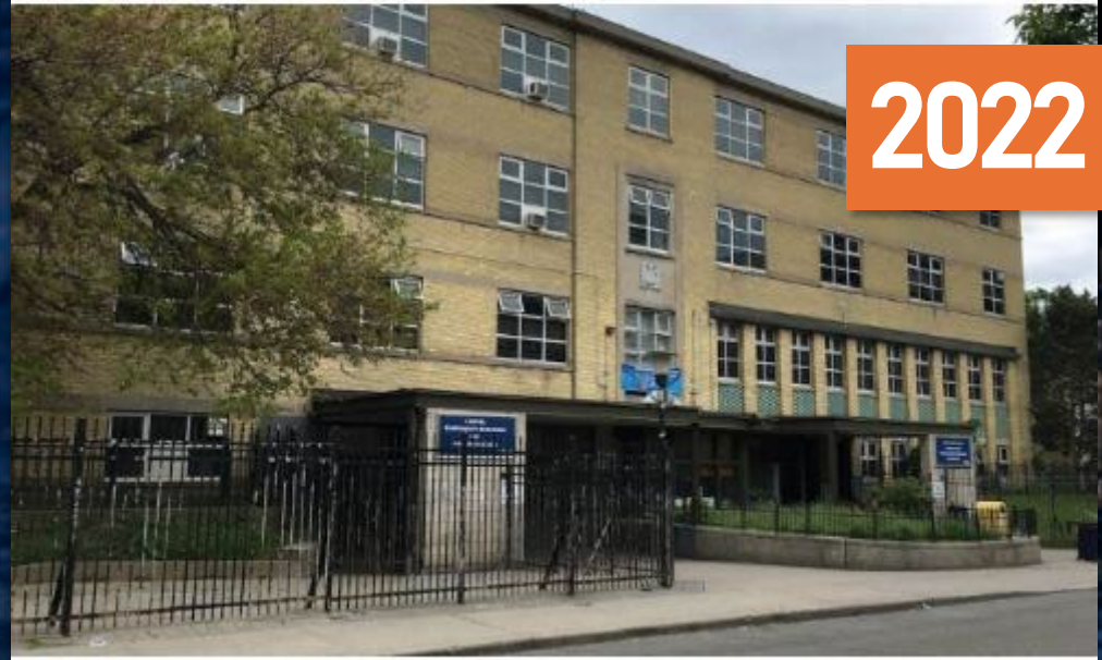
A view of Seaton House, a large homeless shelter in downtown Toronto, in May 2022.
